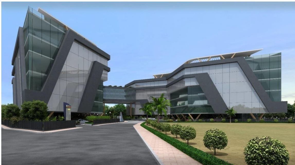
Figure 1 Proposed view of the Business cum Tourism and Cultural Centre at Police Bazar
