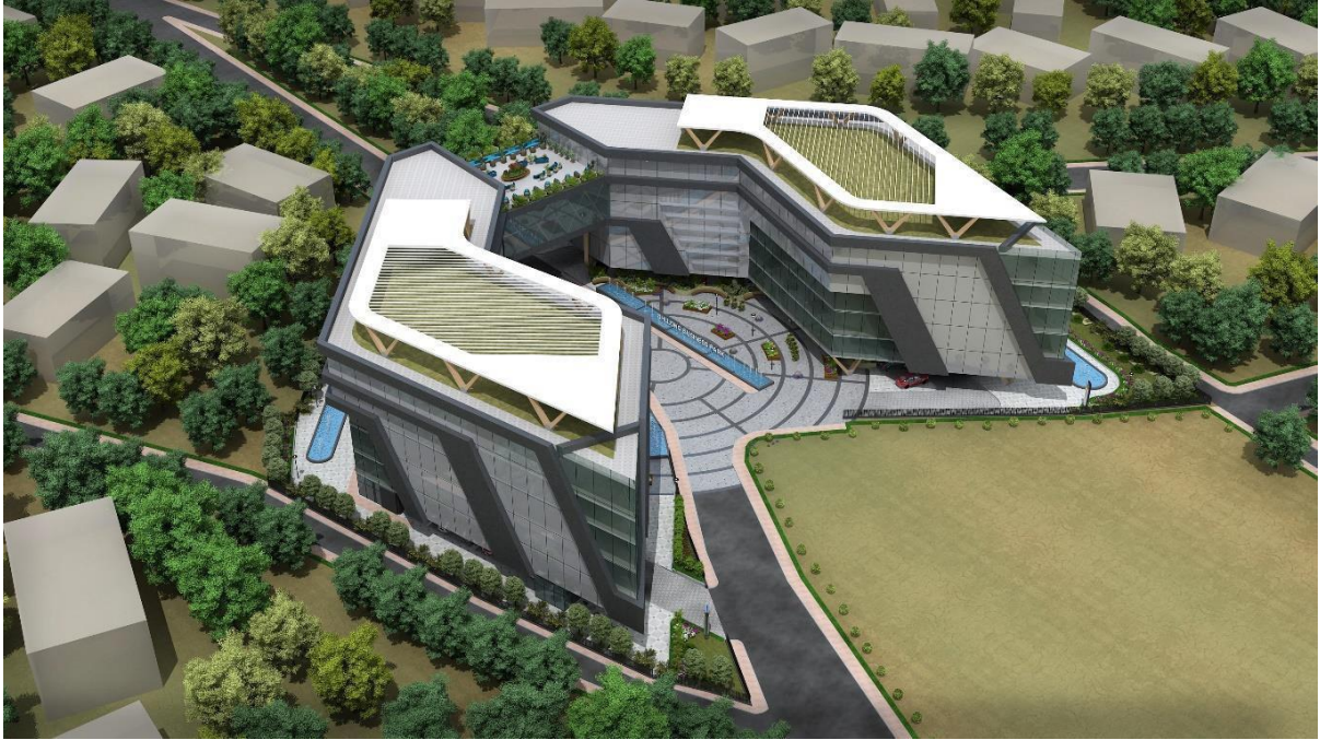
Figure 40 View of the structure from the top
