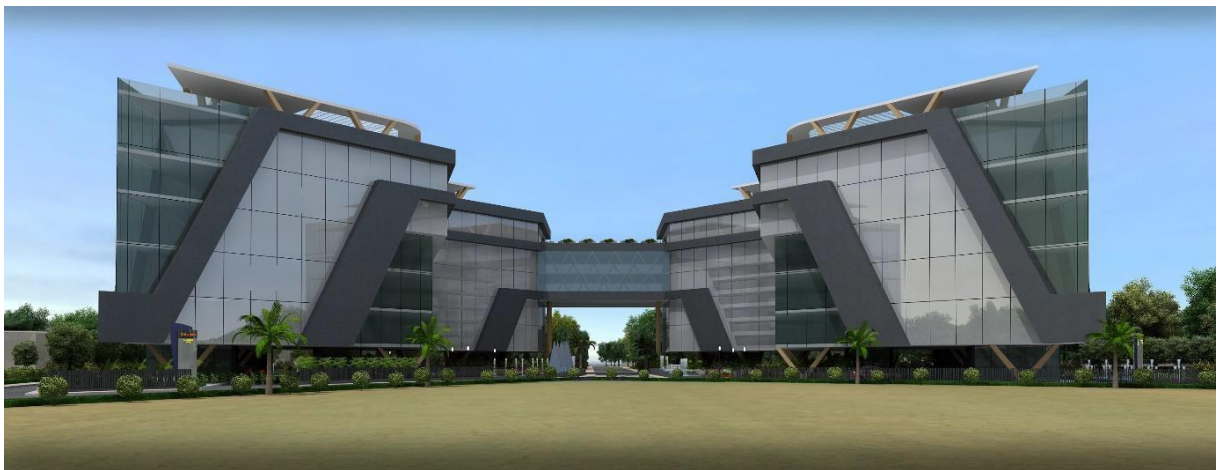
Figure 39 View of the Business cum Tourism and Cultural Centre from the north
